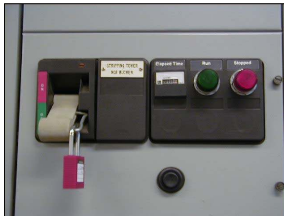
Figure 4 – Example of switch lockout
