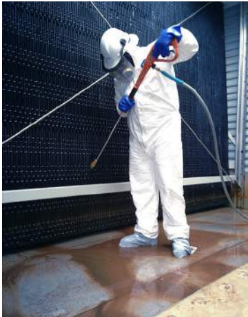
Cooling tower cleaning
